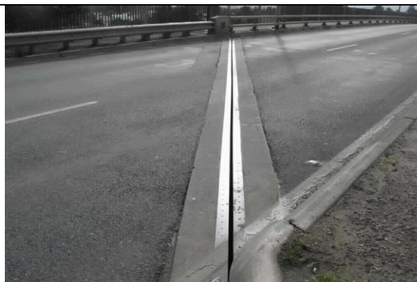
Armoured joint in good condition
