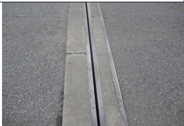
Spalled nosing
