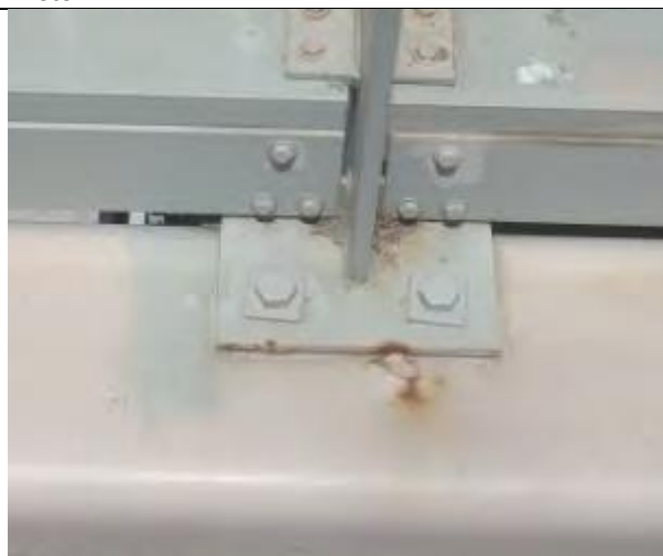
Spot rusting on steel kerb
