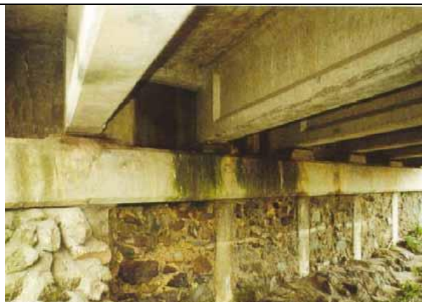
Precast high strength reinforced concrete "I" beams in good condition (VicRoads)
