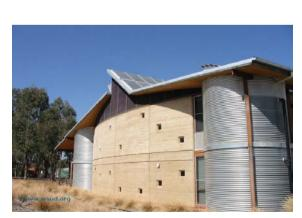
Rainwater Retention tank (above ground)
