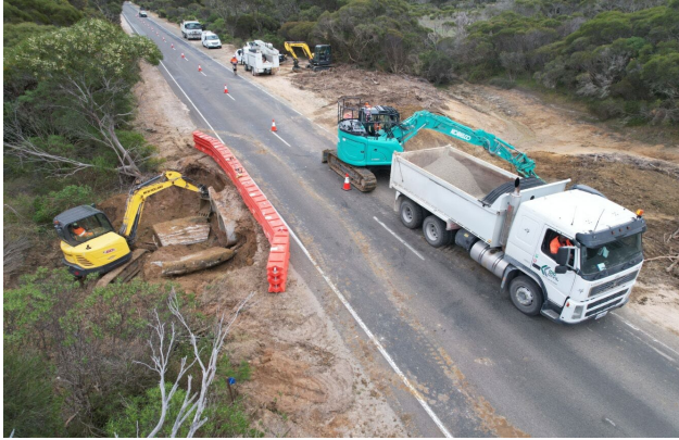
Drainage upgrade works on Hog Bay Road
