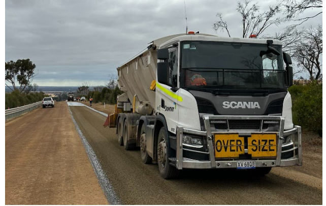
Initial seal installation on the Playford Highway
