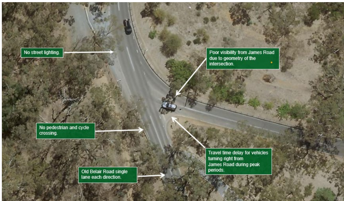
Source: DIT Mitcham Hills Corridor Old Belair Road Upgrades Project Public Works Committee Report
