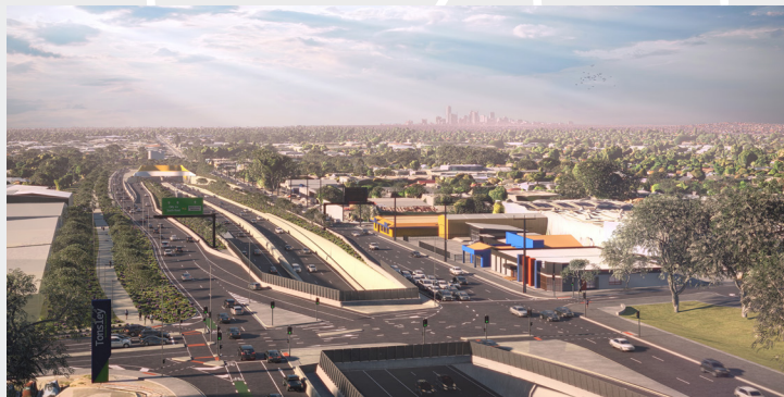
Southern Tunnels entrance / Tonsley Boulevard
