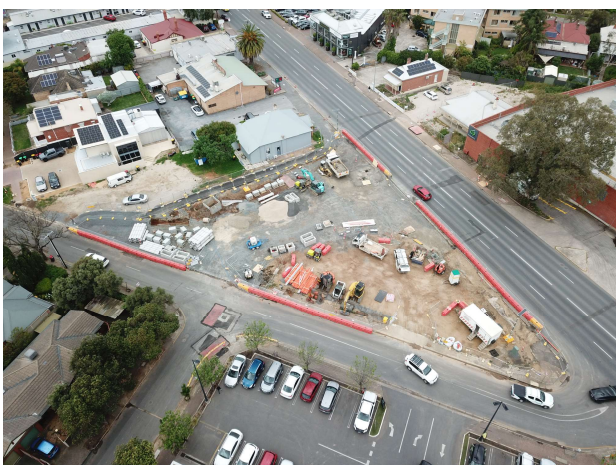
Main Avenue and Glen Osmond Road Junction - November 2022
