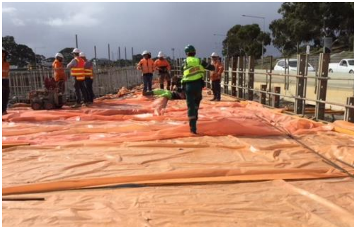
Plastic sheeting covering unidentified hazards underneath
