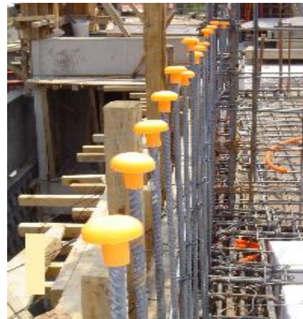
Use correct fitting rebar caps
