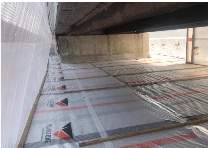
Image 1: Inside of an environmental containment and encapsulation system
