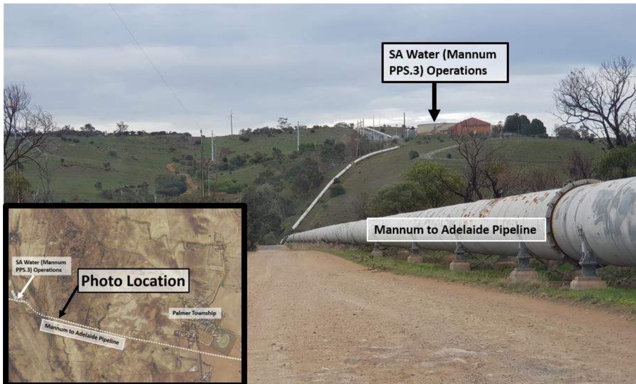
Figure 4. Mannum PPS.3 – site photo taken along Mannum-Adelaide Pipeline access track, facing west-northwest towards existing pump station and, inset, aerial view of photo location (base map source: SAPPA, https://maps.sa.gov.au/SAPPA/ )
