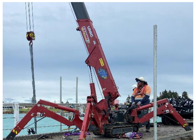
Image: Spider Crane used in decking construction
