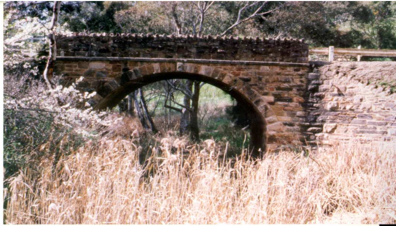
Stone arch bridge, One Tree Hill Road built 1874 - State Heritage Register
