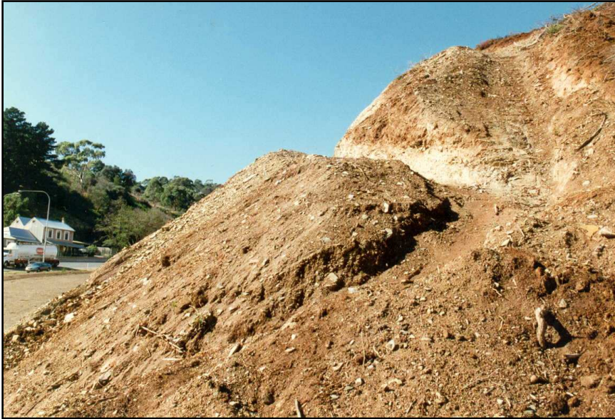
Establish cut off drains around site works
