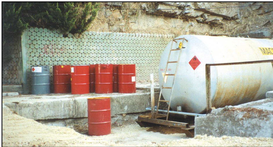
Bund the refuelling area
