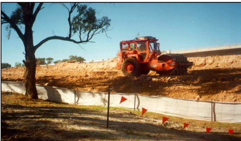
Install silt fences at the toe of batters
