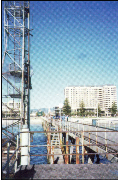
Pile driving – notify affected people if noisy activities will be undertaken
