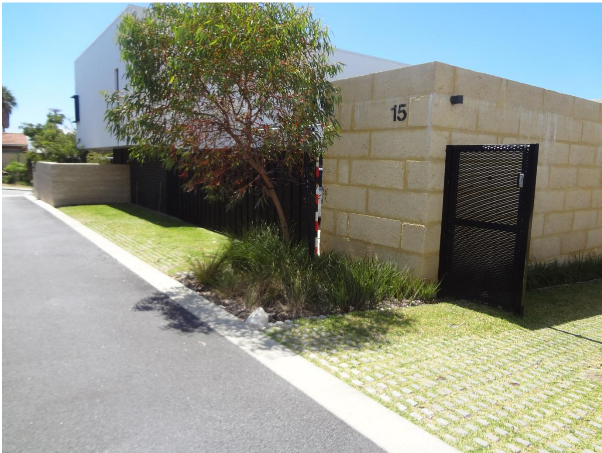
Street verge incorporating WSUD techniques. Source: Water Sensitive SA
