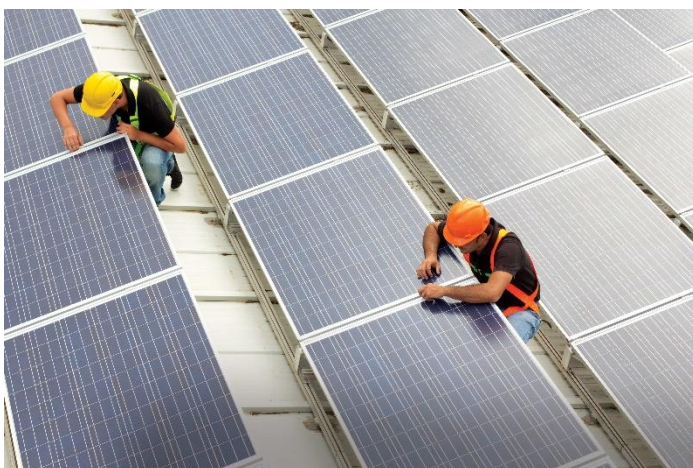
Solar photovoltaic panels being installed. Source: DEW
