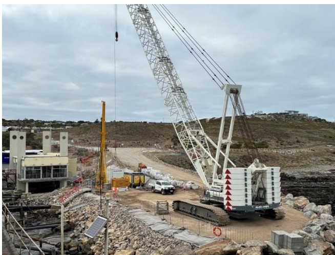
Image 1: Works underway at the Cape Jervis Port precinct
