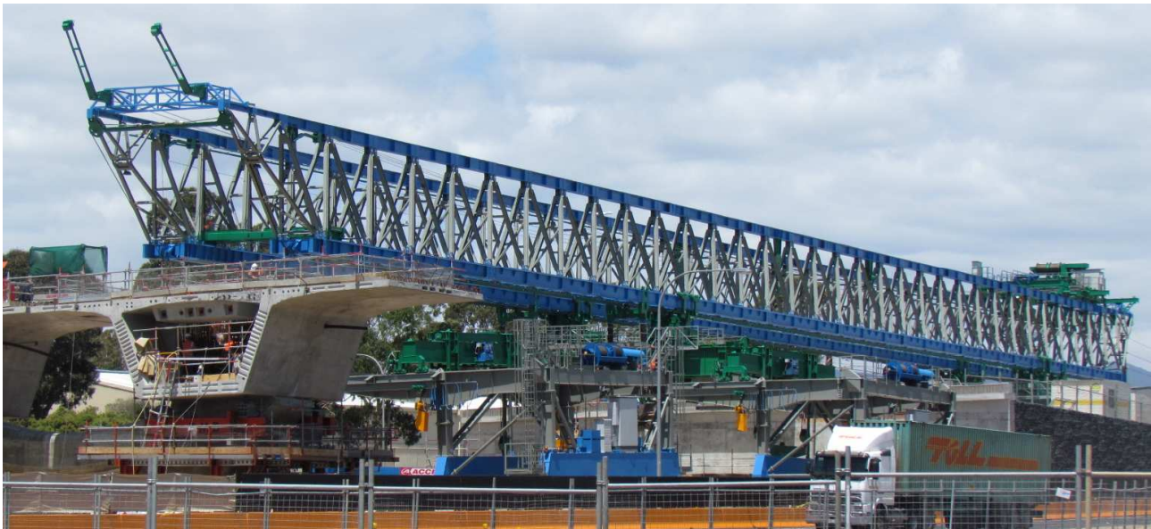
Launching truss on South Road, Regency Park
