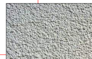
Walls General Trowelled texturecoat on flushed FRC sheeting
