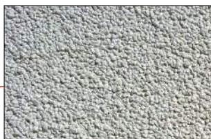
Walls General Trowelled texturecoat on flushed FRC sheeting
