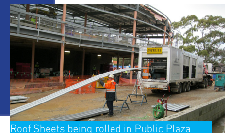
Roof Sheets being rolled in Public Plaza
