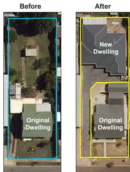
One new dwelling constructed on a 'battle-axe' allotment at the rear of the original dwelling
