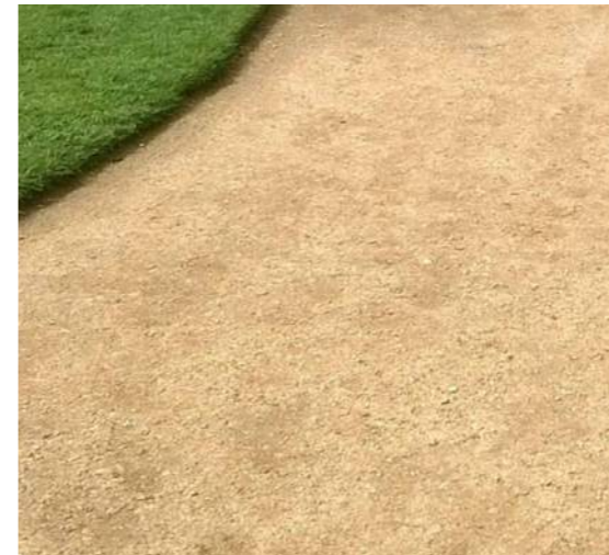
Compacted Gravel (CG)
