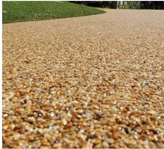
FEATURE Porous Resin Bound Gravel (GR)
