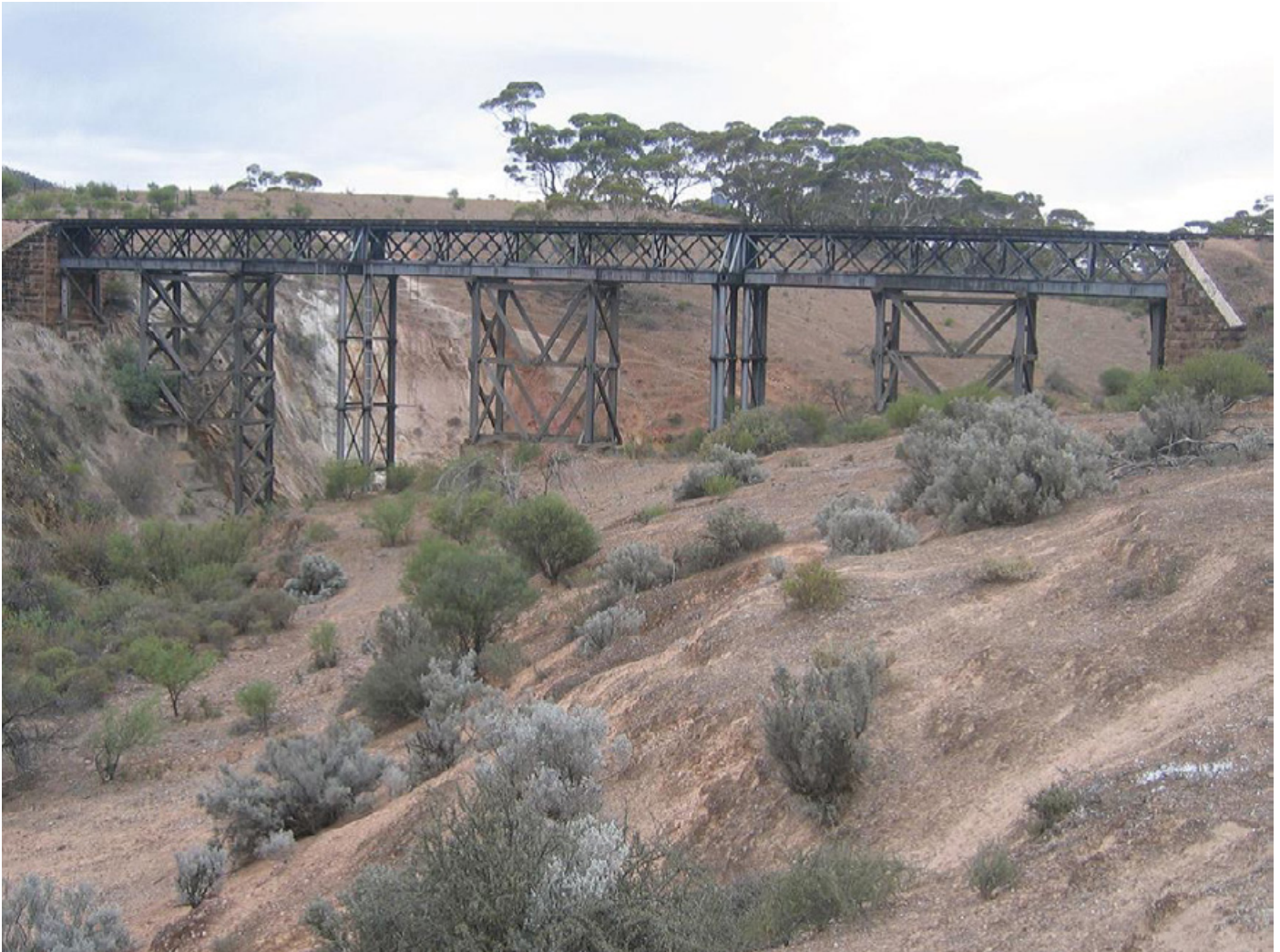
Lattice Bridge; Railway bridge and stone abutments. This is considered a good example of early railway infrastructure.
