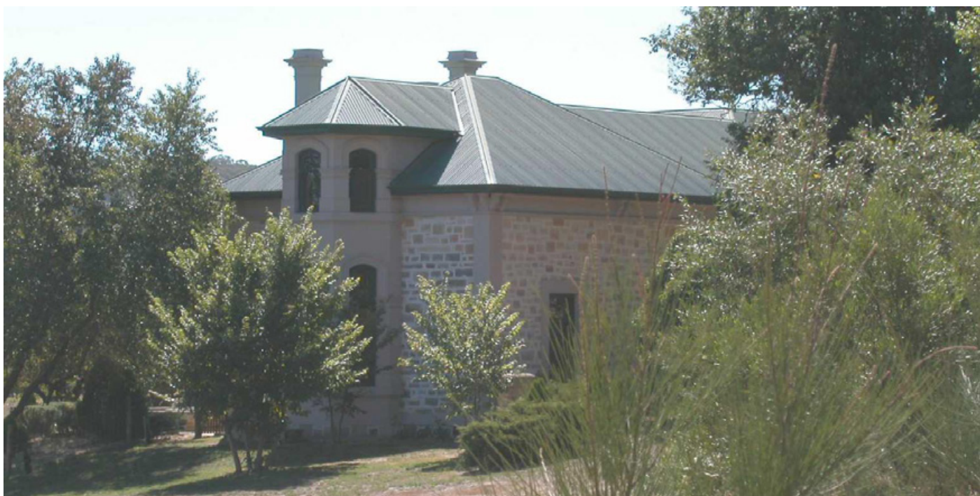
“Warrakilla” House, former Wheatsheaf Inn. The place has strong associations with surveyor George Goyder and notable architect Daniel Garlick”. Photo source: DC Mount Barker Heritage Survey, Part 3: Local Heritage Recommendations: Biggs Flat to Hahndorf, Heritage Online, Anna Pope and Claire Booth, 2004
