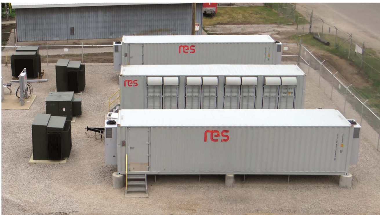
Plate 2-6: Typical layout of containerised system
