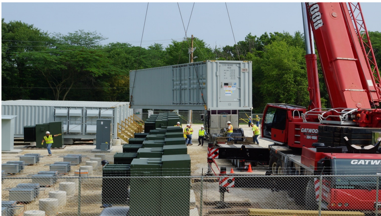
Plate 2-5: Typical construction of BESS
