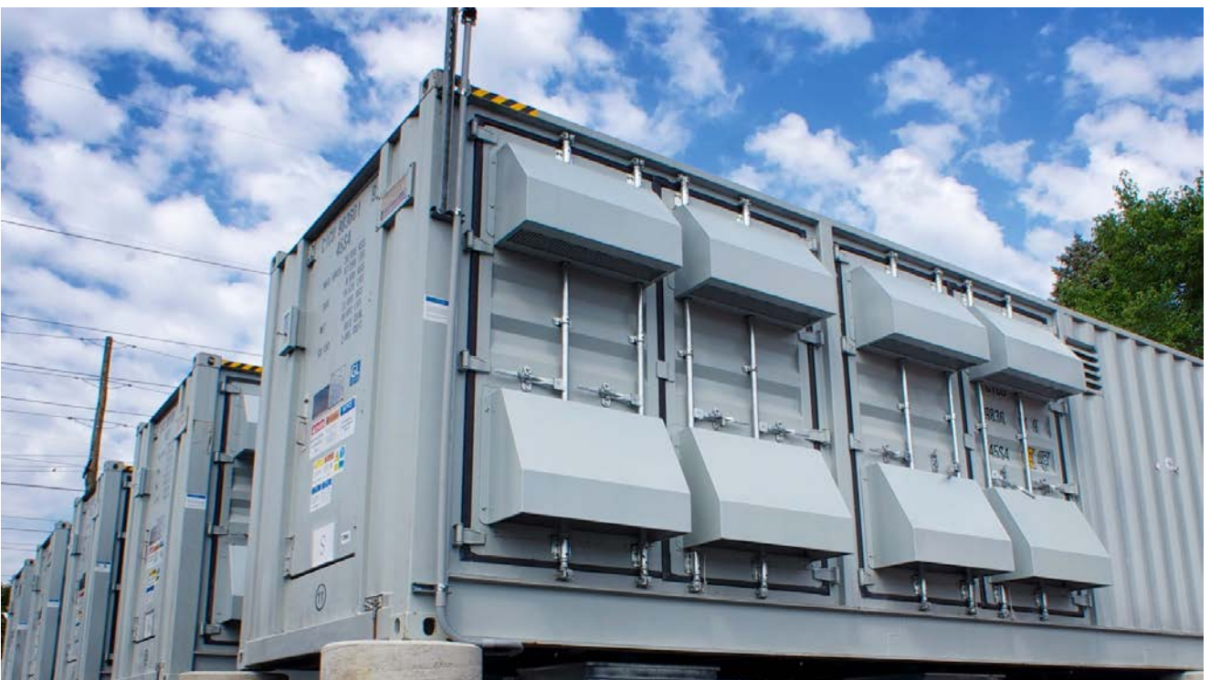
Plate 2-4: Typical containerised system for BESS projects
