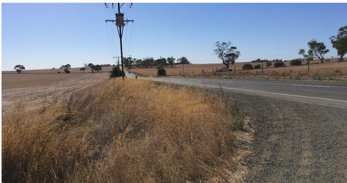
Figure 4 Sight Lines from Power Road to the Eastern Approach of Templers Road
