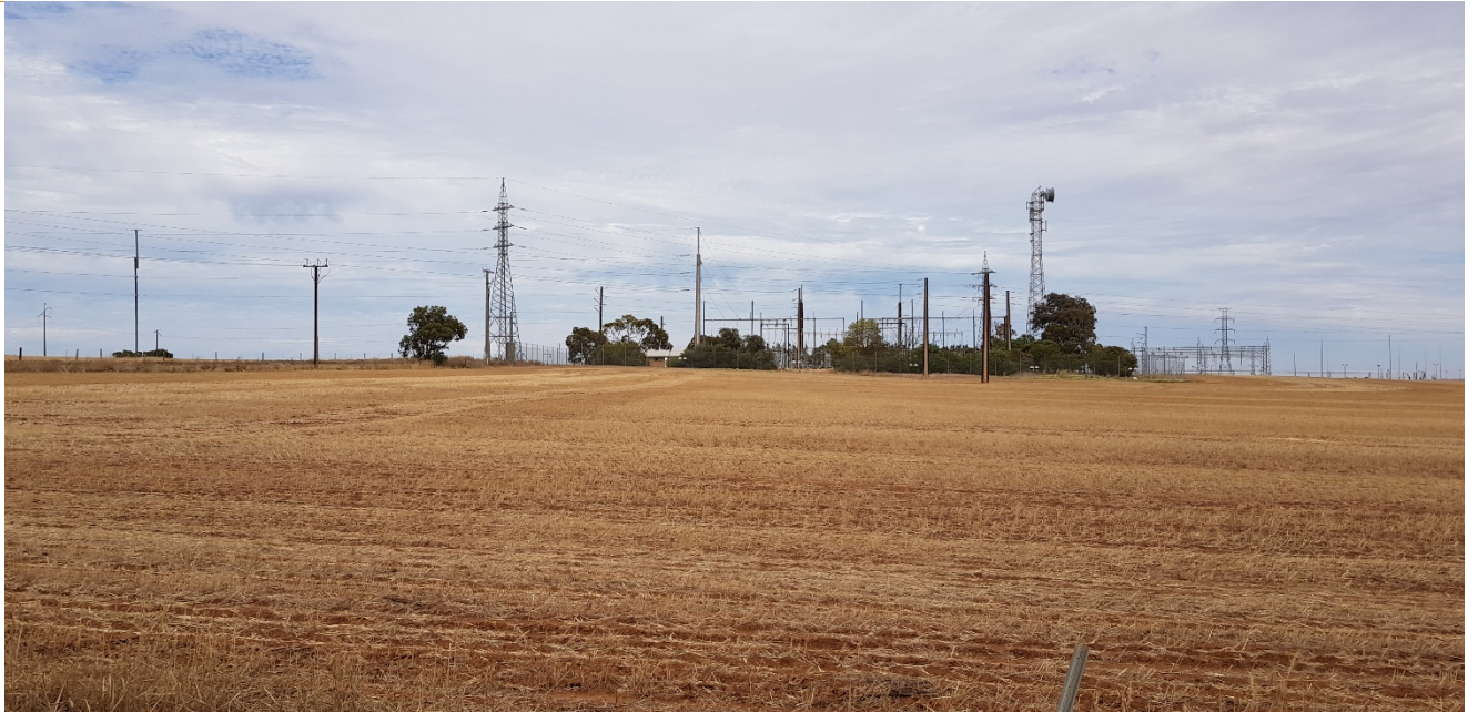
Plate 2-1: View across the Project site, showing Templers substation in the foreground and Templers West substation in the background (Source: RES Australia)
