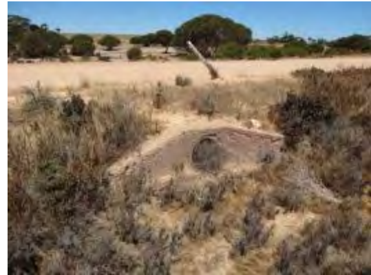
Right: Culvert on Balumbah-Kinnard Rd
