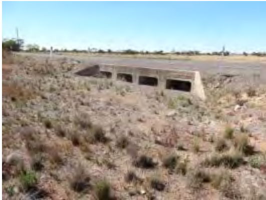
Left: Culvert on Birdseye Highway
