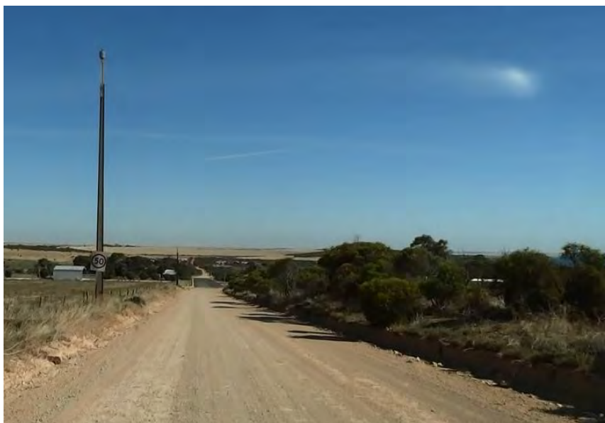
Plate 5-2 Power line parallel to haul road (North Coast Road, Port Neill)
