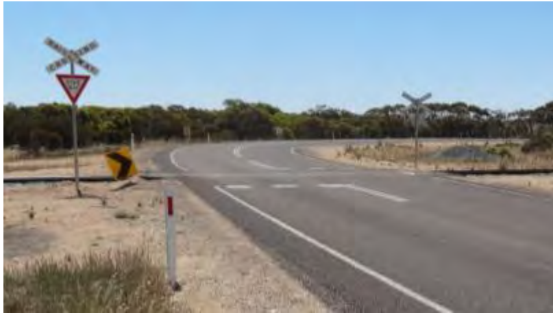
Plate 5-3 Rail crossing on Balumbah-Kinnard Road
