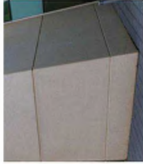
3. BRIGHTON LITE CONCRETE 3a. GRC CLADDING
