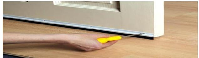
*Acoustic seal being installed on a door*
