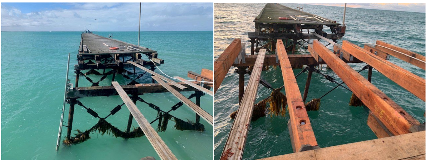
Timber framework refurbishment works at Beachport Jetty.
