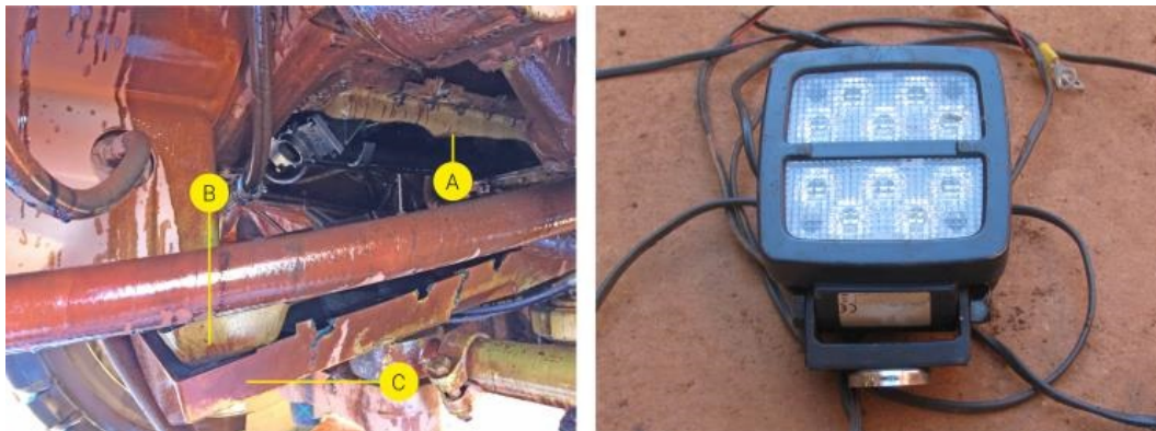
Left: Sump damage, showing the failed sump (A) and the sump remnant (B) that had fallen down into the sump cover (C). Right: LED lamp used to illuminate the work area.
