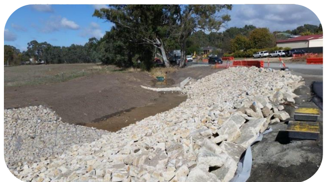
Reuse of crushed concrete on batters at Bald Hills freeway interchange, Mt Barker
