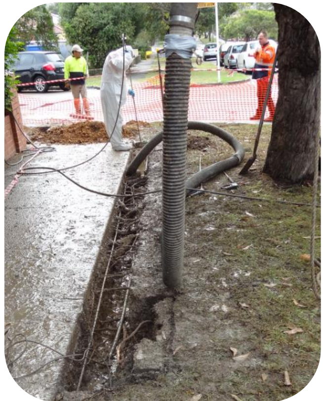
Non destructive digging with correct use of soil bund and vacuum truck
