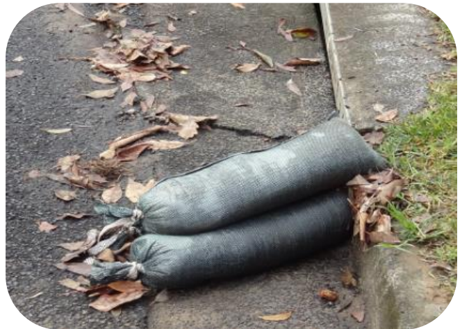
Correctly placed silt socks
