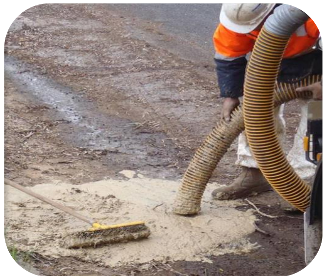
Containing drilling mud during horizontal directional drilling
