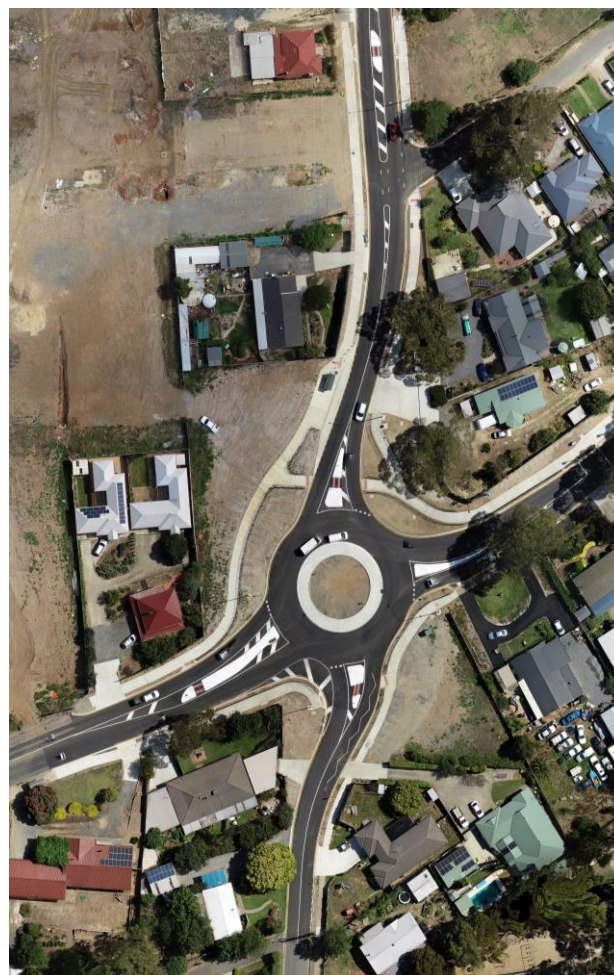
Drone image of the new Nairne Roundabout
