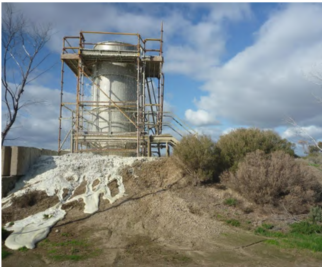
Figure 10. Seawater spilling from a vent connected to an underground seawater pipe. Water runs east along a drainage line into the Coastal Saltmarsh.
