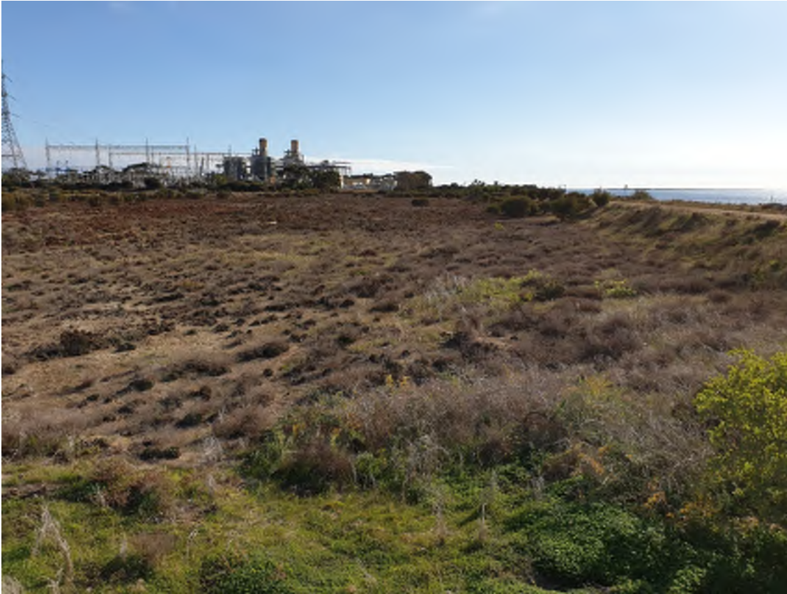
Photo 2.2 View from the centre of the Site, looking north-west, showing the existing Pelican Point Power Station to the south
