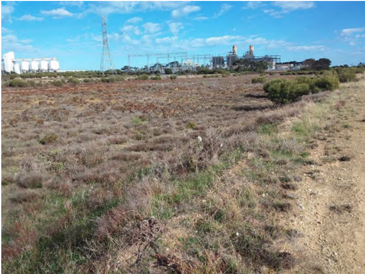
Photo 1 – Gas Turbine Peaker Project site at Pelican Point
