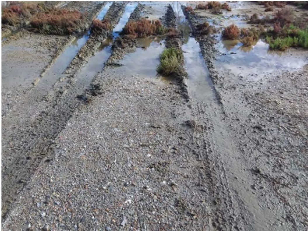
Photo 4: Road section with soft ground condition
