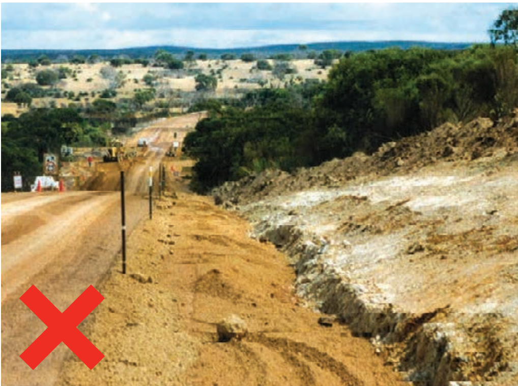
Soil erosion control measures need to be installed
