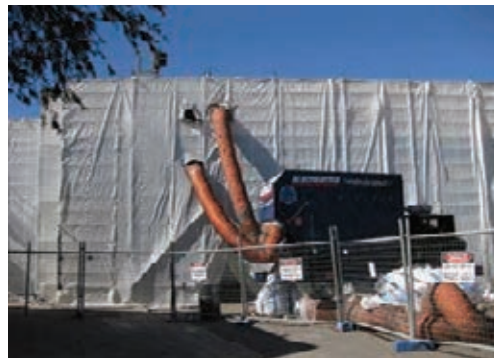
Encapsulation of the Port Adelaide rail bridge during lead paint removal
