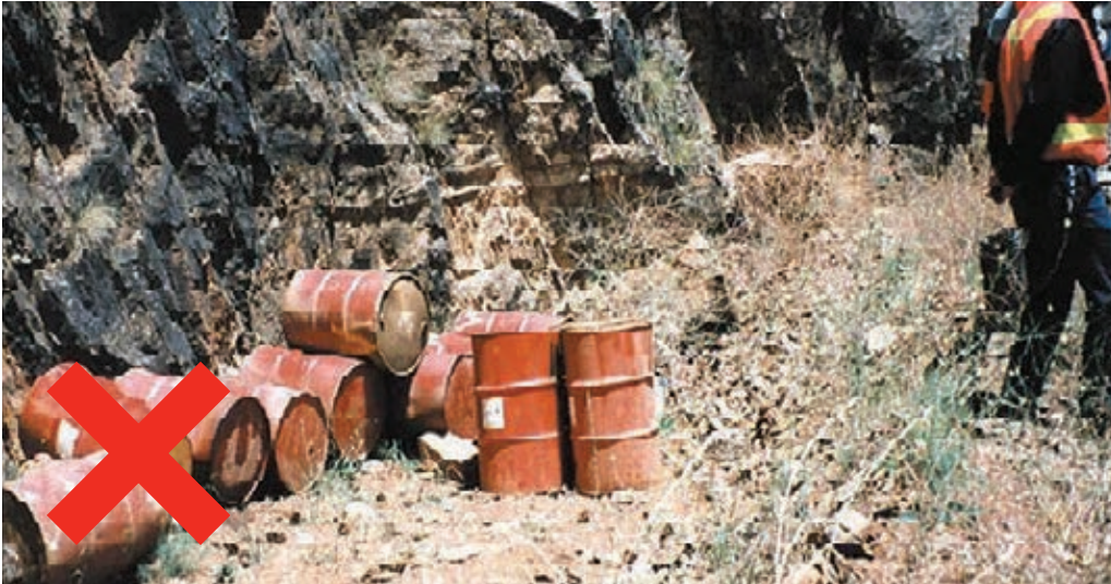
Poor storage of materials
